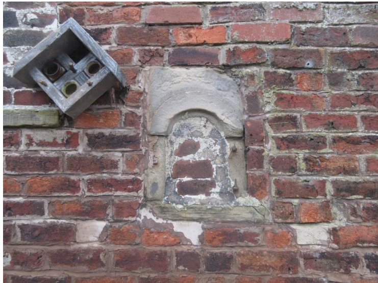
Early shuttered window opening rebuilt into outbuilding.
